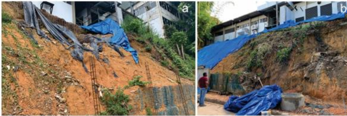
Figure 8 - (a) Moment before part of the slope falls; (b) view from another angle of the slope.
