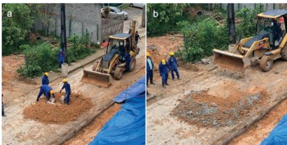
Figure 9 - Soil-cement process; (a) Four 42.5kg bags of Portland CII cement and approximately 4.2m 3 of clay were used; (b) Mixing process between materials.
