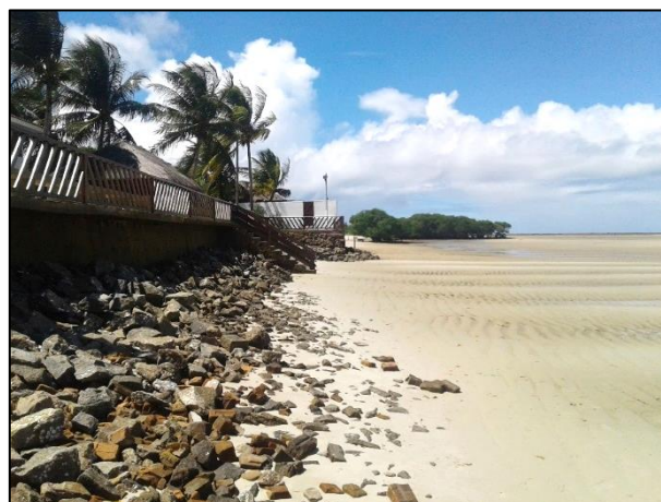
Figure 5 – High vulnerability area: concrete-faced rockfill beach dams for waves overtopping; High post-beach urbanization; and absence of beach during high tide. Source: Author.
