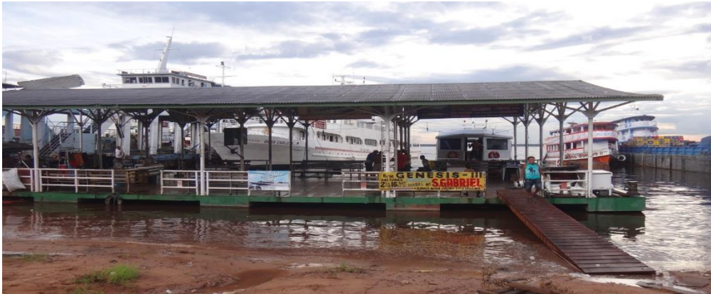
Fig 4: Floating ferry with fingers from behind.
