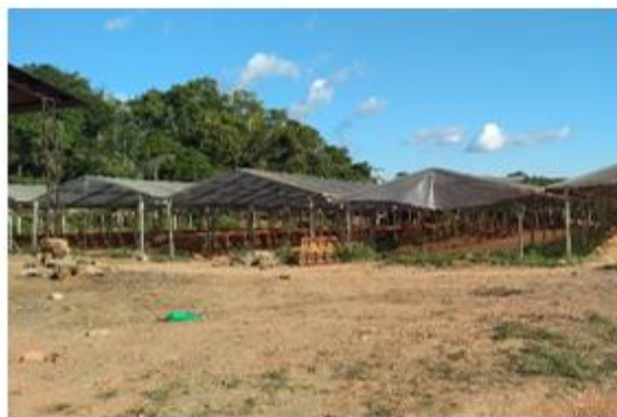
Figure 14: External drying area
