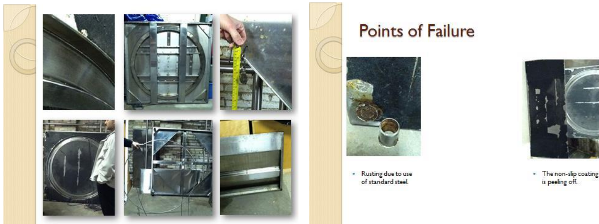
Figure 3: Photos of the old bubble tower and some of the failure point, junior team.
