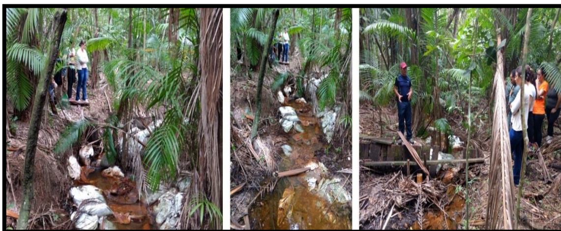
Figure 7. Construction of Mindu Park Containment.
