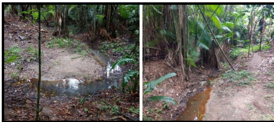
Figure 3. Clearance of the Nanuente of Mindu Municipal Park.
