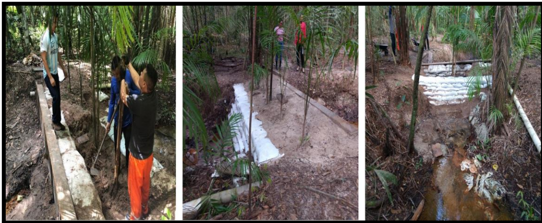
Figure 9. Implementation of sandbags and planting of seedlings in containment.
