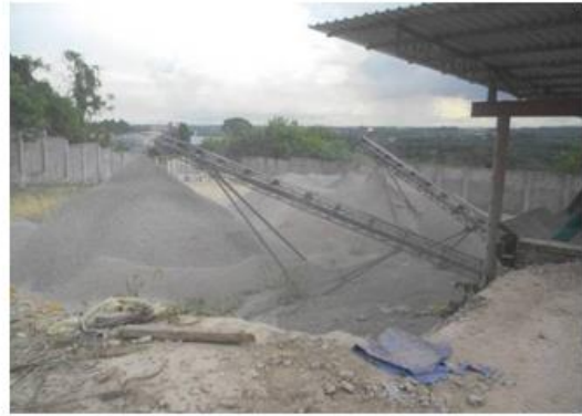
Figure 2. RCD block crushing and sieve separation
