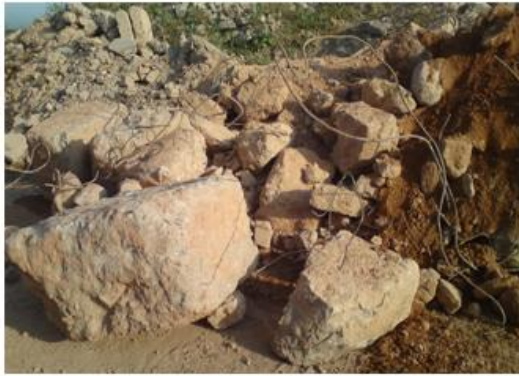
Figure 1. Construction and Demolition Waste Storage - RCD
