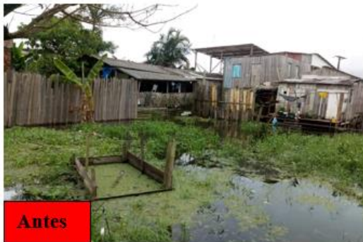
Figure 2: Flooded houses during floods.
