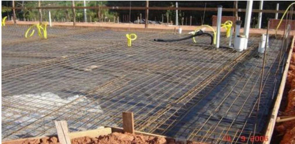
Figure 01: Radier type foundation
