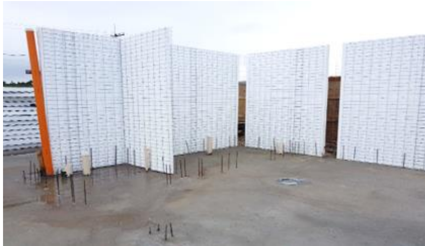
Figure 03: Panel fixed on the start-ups of the radier type foundation
