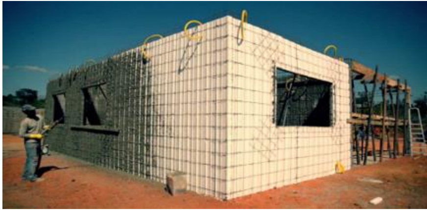
Figure 05: Application of microcement with equipment
