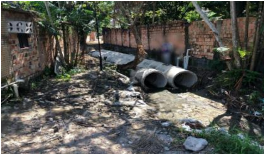
Figure 2: Laying of drainage pipes.
