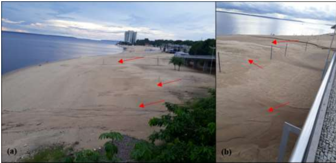
Figure 11: Features found on the landfill surface during low water periods, in 2019 - a) and b) Beach surface presenting, in general, the sandy mass movement features.
