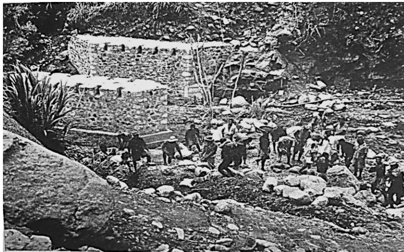
Picture1: The construction of roads and bridges in the Bafut Fandom
