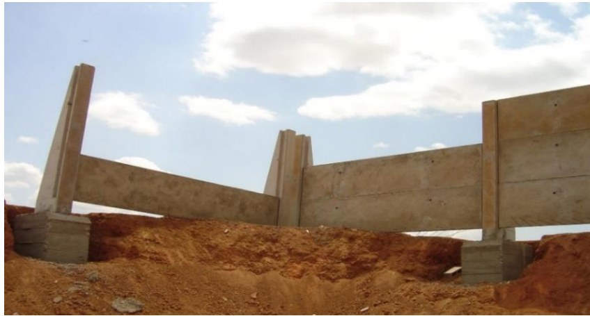
Figure 5 - Assembly of the precast wall of a horizontal silo
