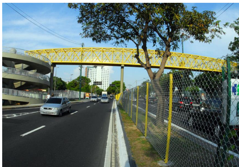
Figure 4. Footbridge Amazonas Shopping. Source: Acrítica.com
