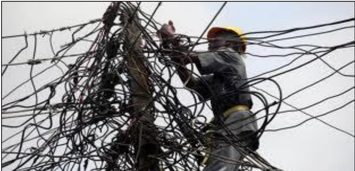
Figure 3: Illustrative photo of an employee of Rede Celpa (Equatorial) cutting off clandestine power on Tv. Humaitá corner with Rua Nova, city of Belém, Pará, Brazil.
