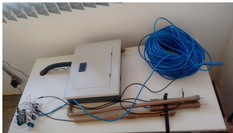
Figure 6 - Installed System with 100 Meters of CAT E6 Cable. Source: The Author, (2021).
