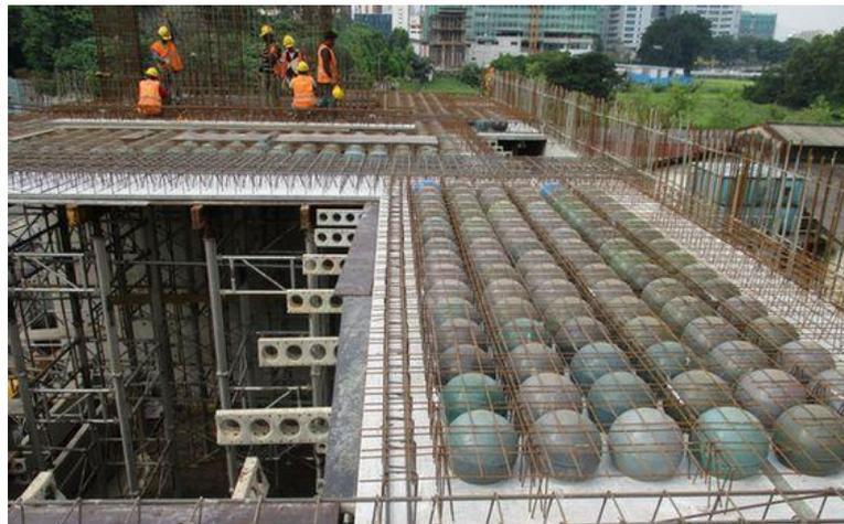
Figure 1: Bubble deck slab system at the construction site
