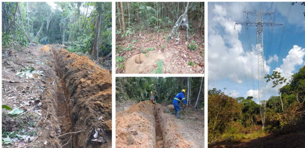
Picture 8. Execution of the activities on site.
