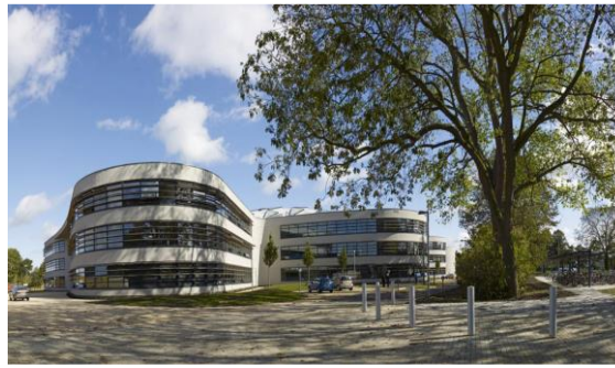
Figure 3 - Facade of the Institution
