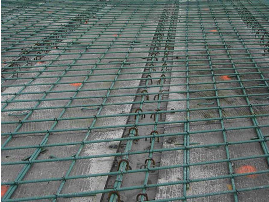
Figure 19 Top layer of reinforcing steel in place on top of partial-depth panels (WSDOT)
