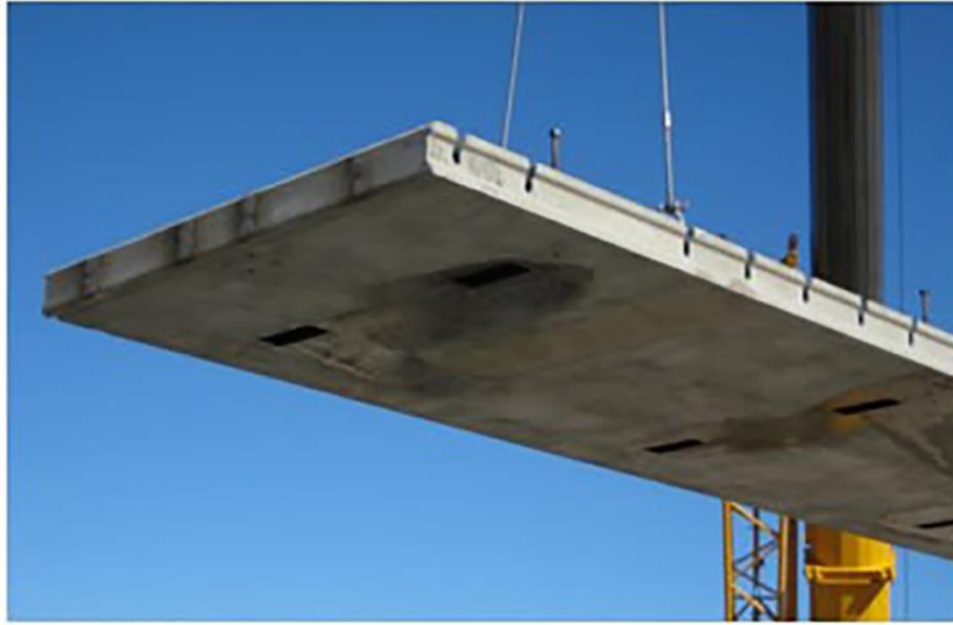
Figure 13 Full-depth Deck Panels ( https://www.fhwa.dot.gov/bridge/abc/prefab_def.cfm )
