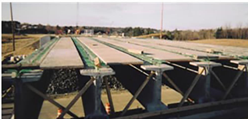
Figure 12 Partial-depth Deck Panels ( https://www.fhwa.dot.gov/bridge/abc/prefab_def.cfm )
