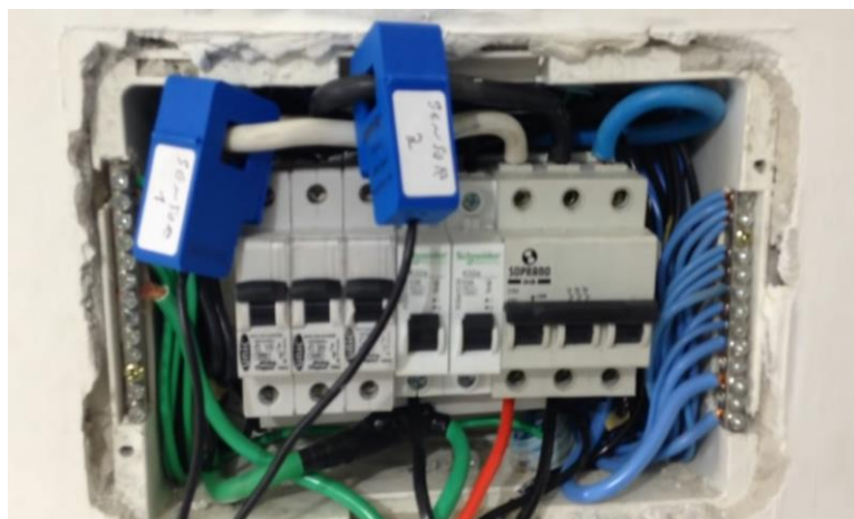
Figure 3. Integration of current sensors to the residential distribution board.
