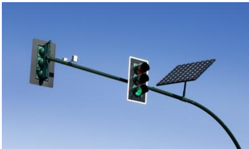
Figure 3 - Traffic light with photovoltaic power system in Manaus
