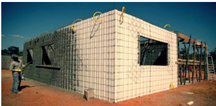
Figure 05: Application of microcement with equipment
