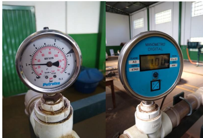
Figure 2. Bourdon type digital and analog pressure gauge.
