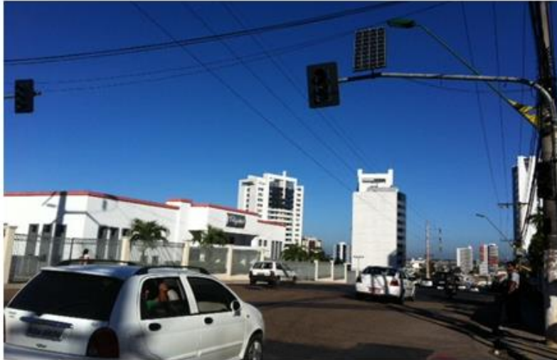
Figure 2 - Traffic light with photovoltaic power system in Manaus
