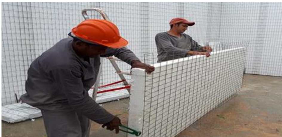
Figure 02: Stapler for Mooring of Panels in The Starts
