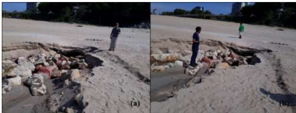
Figure 4: Features found on the transition surface of the embankment and natural beach, during the drought periods, in 2018 - a and b) Erosions with the appearance of the substrate rocks, approximately 2 meters wide, and 40 cm deep.
