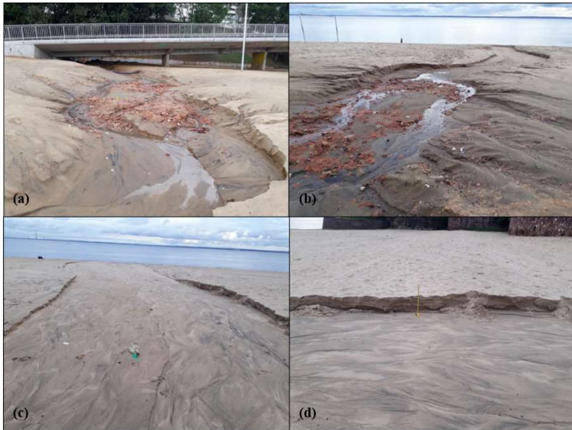
Figure 9: Features found on the landfill surface during low water periods, in 2019 - Features of sandy movement due to rain. Photo a) shows the sediments from the beach, and in photos b and c) show the sediments towards the river. Photo d) illustrates the depth of approximately 30 cm of the path caused by the transport of particles.
