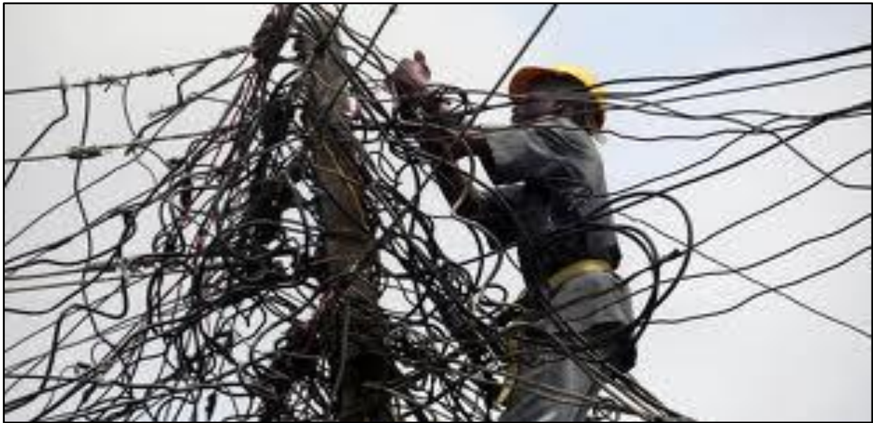
Figure 3: Illustrative photo of an employee of Rede Celpa (Equatorial) cutting off clandestine power on Tv. Humaitá corner with Rua Nova, city of Belém, Pará, Brazil.
